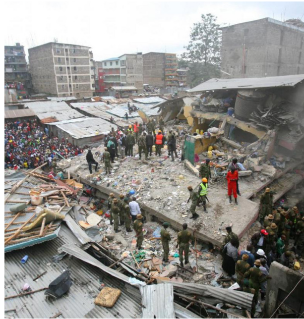
Figure 3: Collapse of a Six-story Residential Building in Huruma, Nairobi
