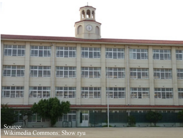
Honjo Elementary School, Kobe: Typical Japanese school buildings are low rise moment resisting reinforced concrete frames with shear walls.
