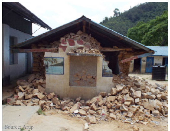
Damaged stone masonry school in Lalitpur, Nepal
