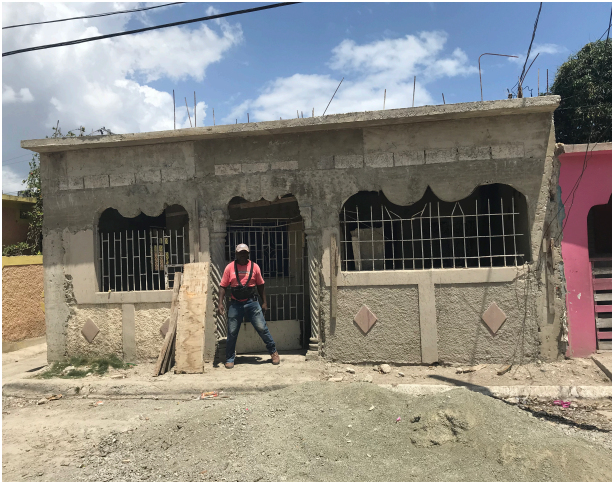
Photos 4 and 5: These photos show a conversion to a slab roof. The practitioner (left) proudly showed the team around. In the photo on the right you can clearly see the addition of a ring beam. You can also see the addition of columns in places where there were previously none. Adding columns like this seems quite common when houses are expanded. Corners and intersections are often cut out and a column added as a retrofit measure. Despite correctly calling them “stiffeners”, most practitioners interviewed believed their main role was to better support the slab rather than help to confine the wall.
