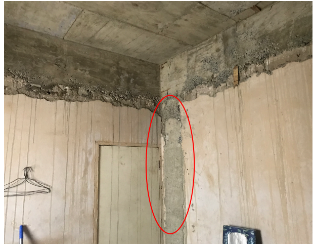
Photos 4 and 5: These photos show a conversion to a slab roof. The practitioner (left) proudly showed the team around. In the photo on the right you can clearly see the addition of a ring beam. You can also see the addition of columns in places where there were previously none. Adding columns like this seems quite common when houses are expanded. Corners and intersections are often cut out and a column added as a retrofit measure. Despite correctly calling them “stiffeners”, most practitioners interviewed believed their main role was to better support the slab rather than help to confine the wall.
