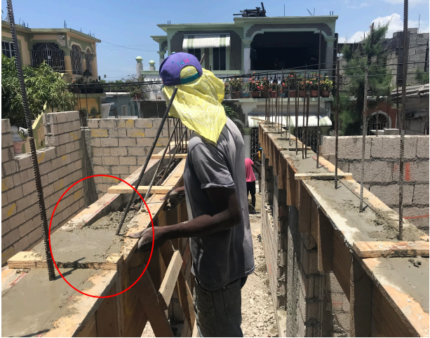
Photo 13: Less than 20% of the construction sites visited mixed their concrete mechanically. In this photo, concrete is being well compacted but is too wet. Aggregate will sink to the bottom severely affecting the final strength. There were no observed instances of concrete being cured.
