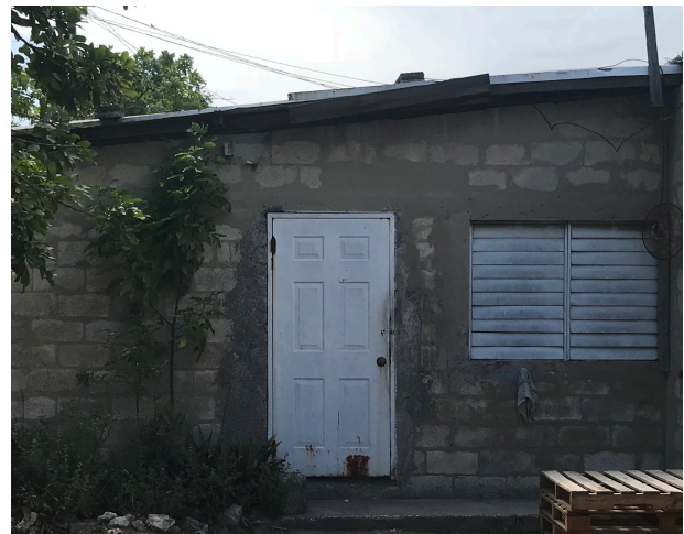
Photos 11 and 12: Zinc roofs were a mix of single slope, double slope and hipped frame. As seen in the picture, houses with single slopes were often very flat. Few if any galvanized hurricane straps were seen although they are reported to be more common now. Rafters are either directly placed on walls or nailed to a wooden top plate attached to the belt beam. The top plate is attached with J-bolts or rebar left over from the vertical reinforcement.
