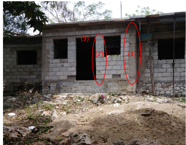
Photo 8: In this example, corner stiffeners are large (1) while other parts of the house go unreinforced. It's likely there are too many openings in the central front wall. The single block piers beside the door (2) would likely fall out of plane during an earthquake and the thin tie beam would be unsupported (3). Once this wall is compromised, so is the rest of the house.
