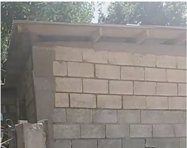
Photos 11 and 12: Zinc roofs were a mix of single slope, double slope and hipped frame. As seen in the picture, houses with single slopes were often very flat. Few if any galvanized hurricane straps were seen although they are reported to be more common now. Rafters are either directly placed on walls or nailed to a wooden top plate attached to the belt beam. The top plate is attached with J-bolts or rebar left over from the vertical reinforcement.
